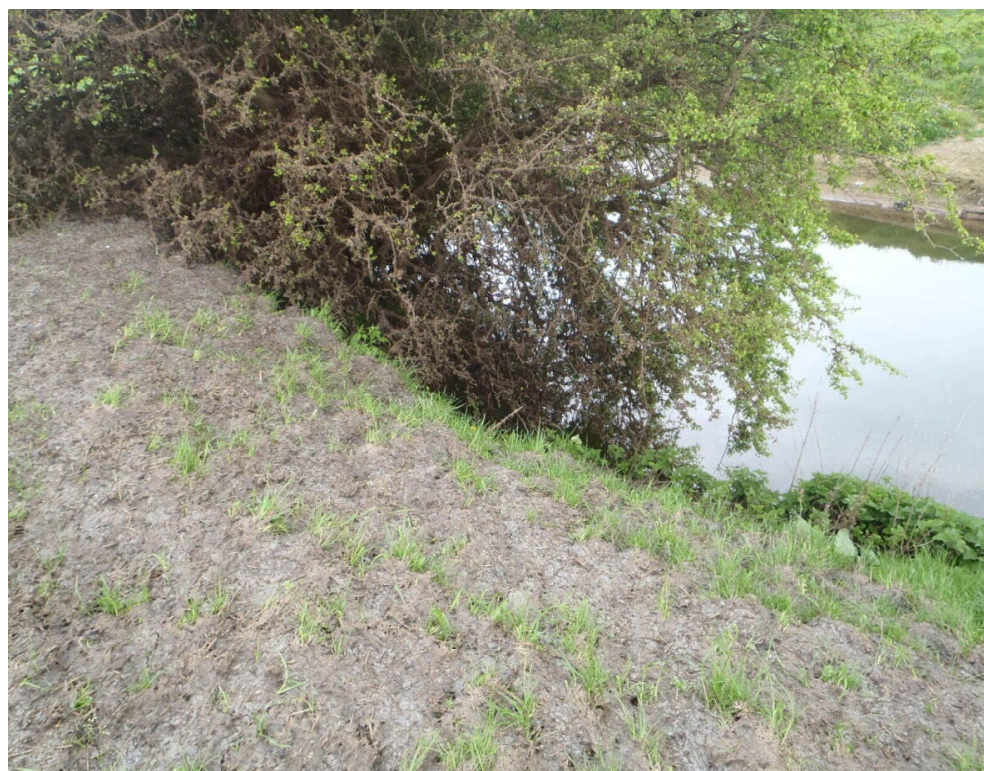
Slurry spread too close to a river (minimum is 10 metres) or 6 metres if using precision equipment
